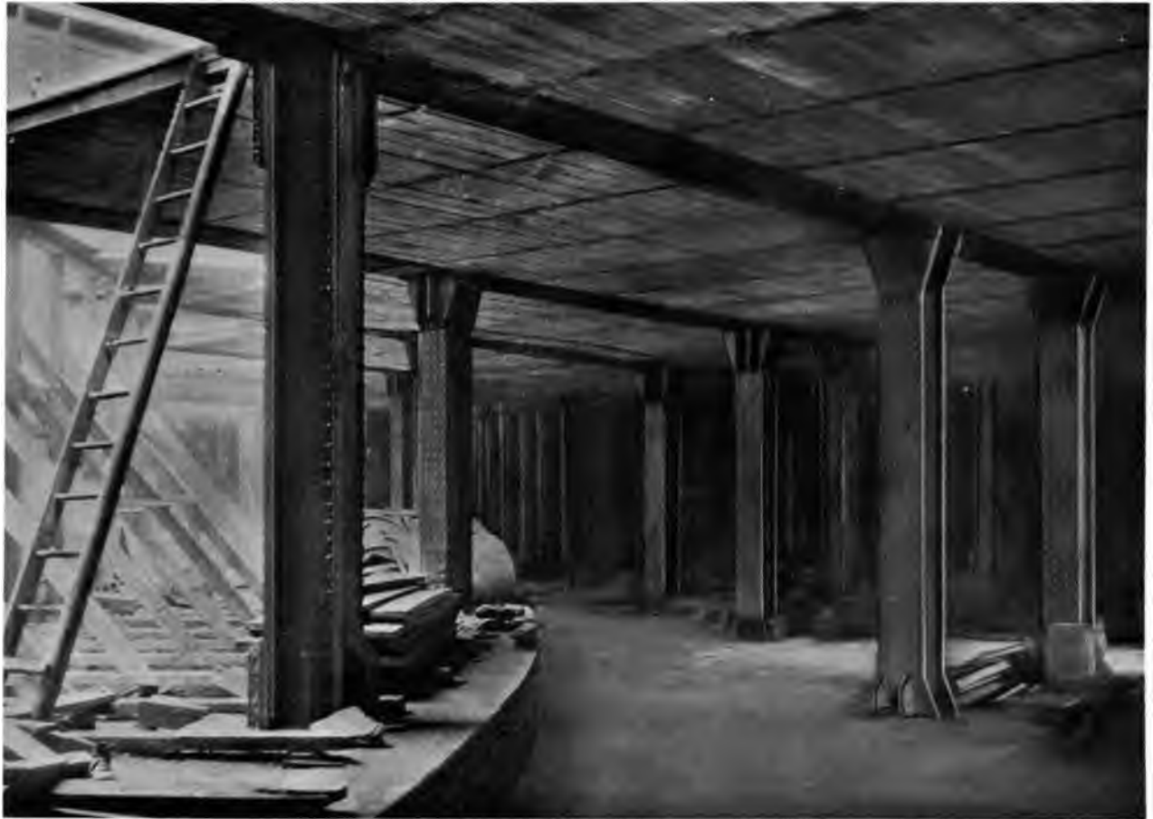
COLUMNS OF HOTEL BELMONT, PASSING THROUGH SUBWAY AT 42D STREET AND PARK AVENUE
